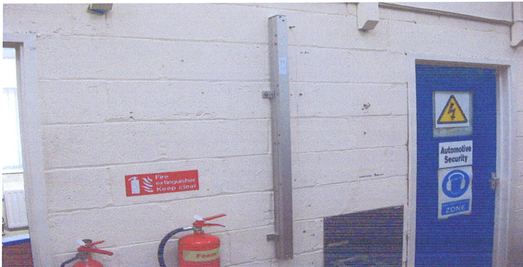
Ladder mounted on breeze block wall.
